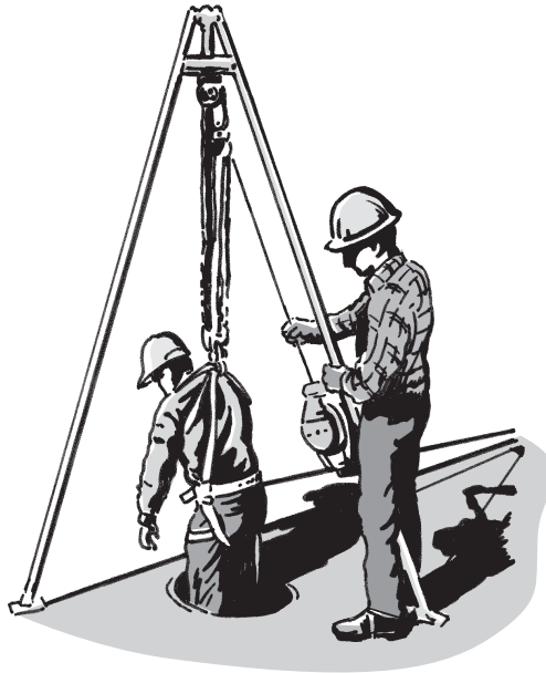
Illustration 3 Retrieval Equipment in Use
